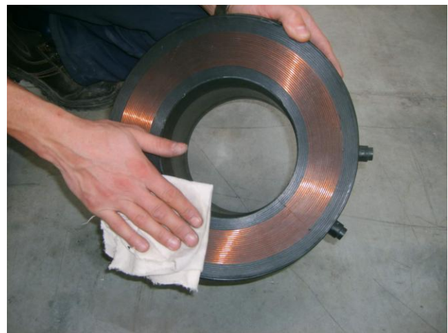
BEFORE WELDING IT IS RECOMMENDED TO CLEAN THE FUSION ZONE ON THE SADDLE AS SHOWN IN PREVIOUS STEP
