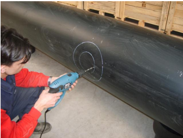
DRILL A 3/8" HOLE INSIDE THE OUTLET LOCATION
