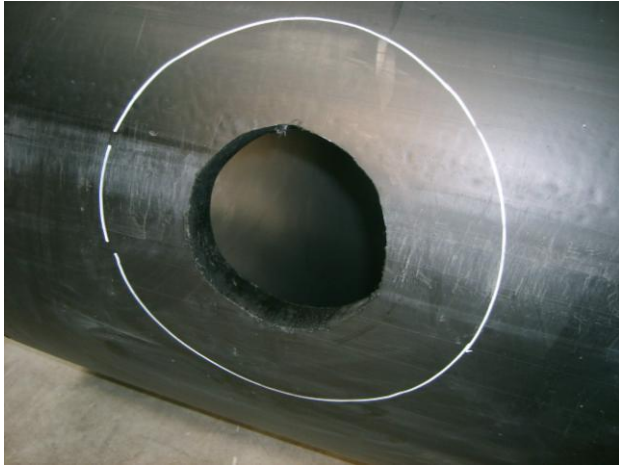
SADDLE LOCATION READY FOR PREPARATION
