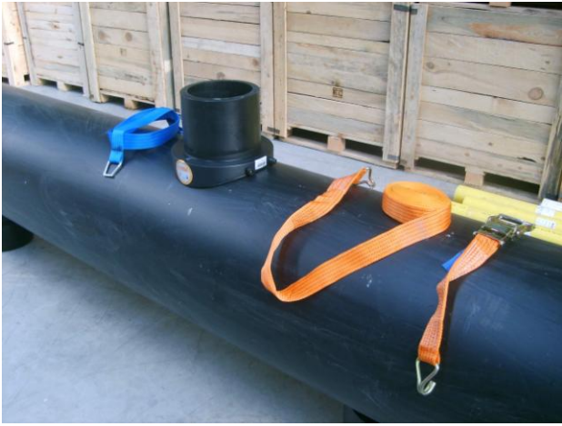
EF SADDLE & HOLD-DOWN HARDWARE BEFORE WELDING
