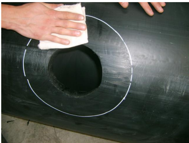
CLEAN SCRAPED AREA WITH ISOPROPYL ALCOHOL(AT LEAST 90%) USING A CLEAN LINT-FREE COTTON CLOTH
