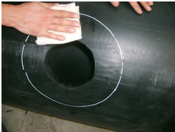
Clean the area that you were scraped before with an appropriate chemical. (Trichloroethone or pure alcohol)
